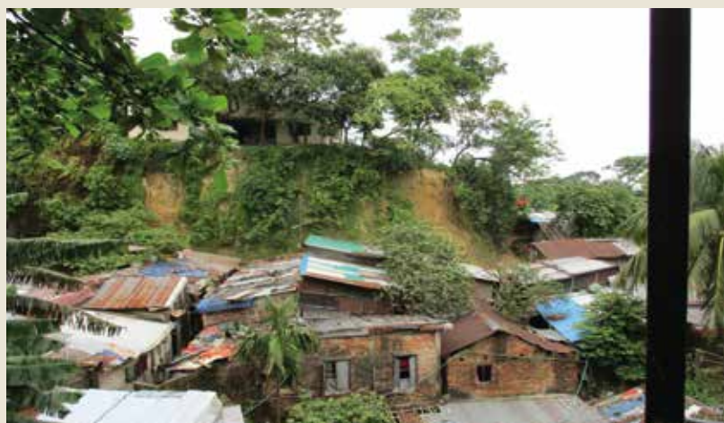
Unsafe dwelling of new migrants in hill slopes
