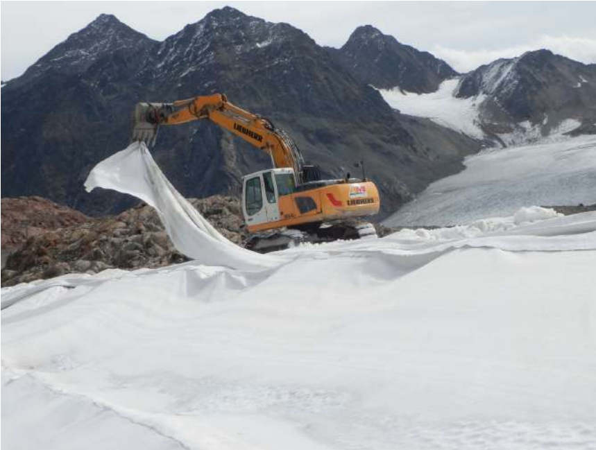
Figure 9.2. A worker uses a digger for removing some textiles in late summer 2015. © Herta Nöbauer.
